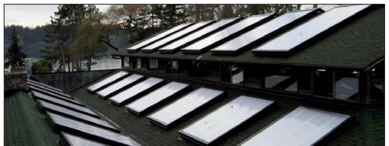
After: IntelaSun® provides control of light transmission, glare, and solar heat gain.
