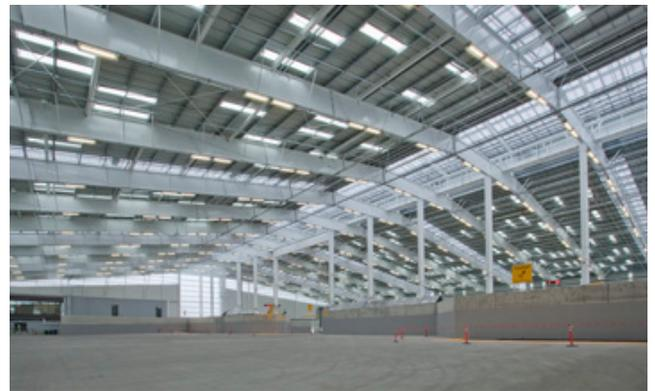
The Quadwall system is an assembly of two independent translucent insulated panels, resulting in one integrated, high-performance daylighting system. Quadwall is the only system that can provide indefinite building envelope protection with its advanced RST – Removable Skin Technology.
