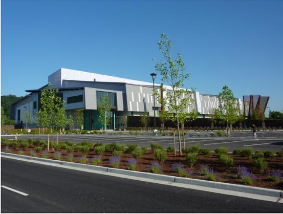
Scalable, the Quadwall system can be configured with additional insulation, FM-rated Class A or B fire-rated roof assembly (chosen for the South Transfer Station), sound reduction, dynamic shading, additional structural performance or even military forced entry resistance. Joined by a mechanically interlocking connection, the dry-glazed Quadwall system eliminates the need for vulnerable adhesives, adding durability, as well as even light distribution with the system's tight-cell technology.
